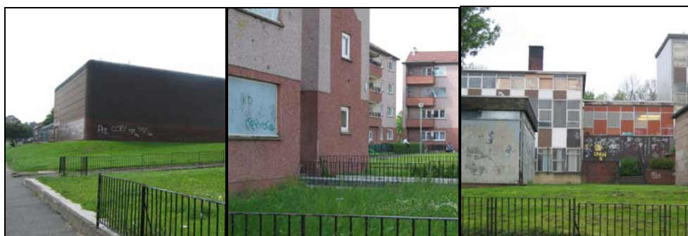
Community centre, Housing in Ruchazie; Ruchazie Primary School
