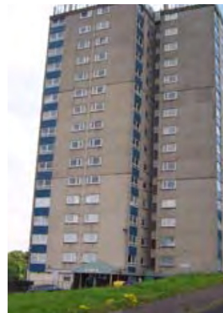
Paisley Tower Block
